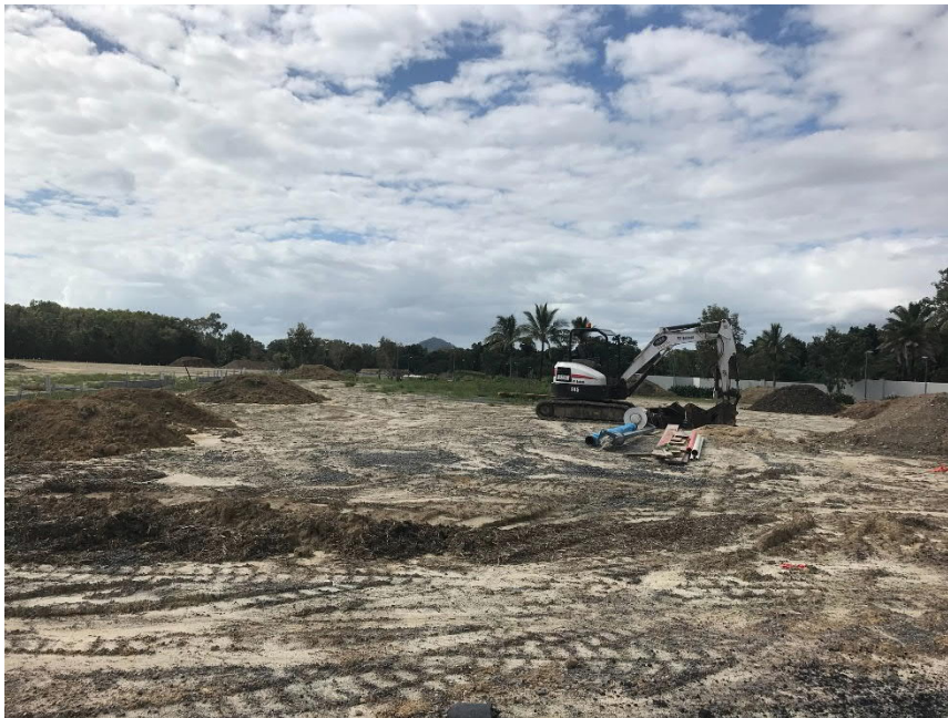
Photograph 1: General Appearance Lot 5, Argentia, Palm Cove
